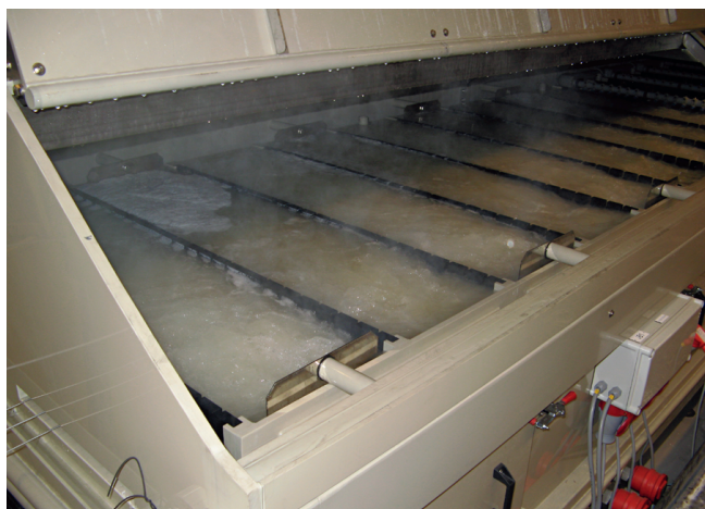
View of cleaning plant.
