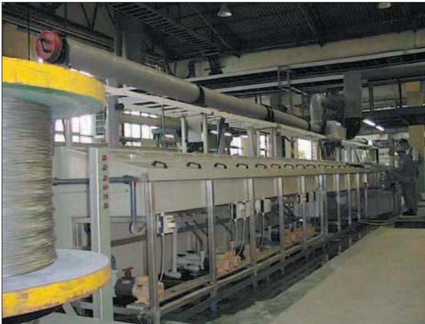
View of plating plant
